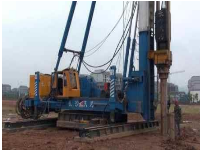
Fig 16: Hydraulic Pile Driving
