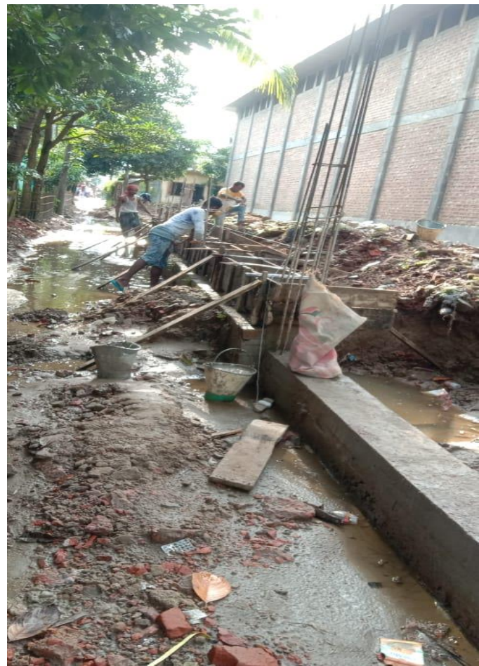
RIVER SIDE BOUNDARY WALL WORKS INCLUDING PRE-CAST PILE AT SACHNA ,JAMALGANJ GOVT. FOOD GO-DOWN
